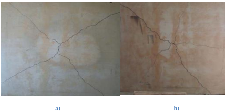
Figure 2.12 Crack pattern, from (Blanco, 2013)
