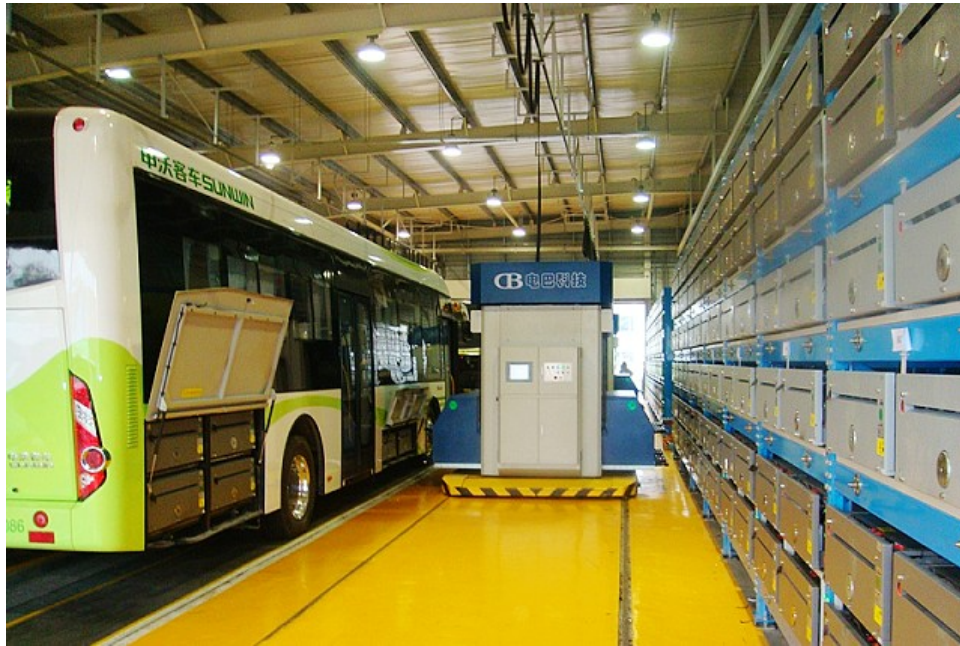
Figure 11 Battery swapping stations for electric busses
