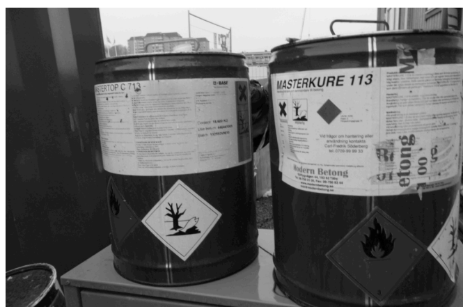
Figure 21. Chemical containers placed outside of the hazardous waste collection safe, observed during a field visit.
