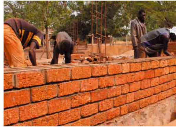
Adobe earth walls
