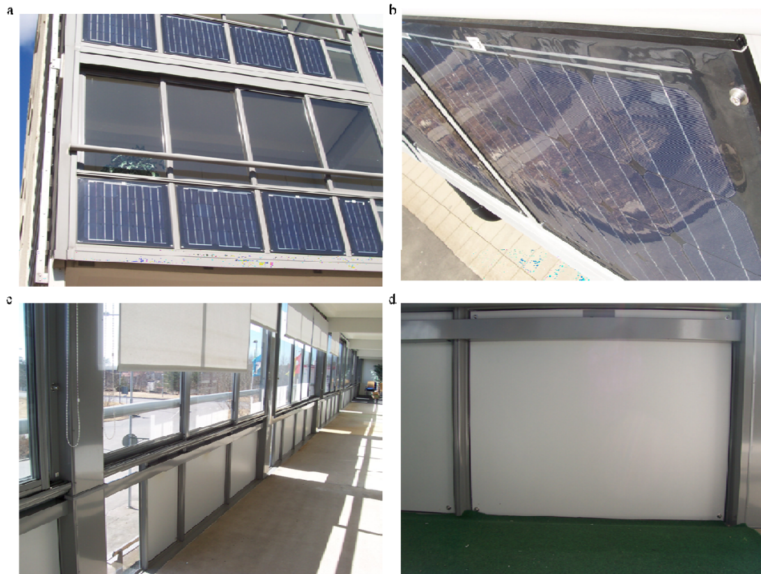
Figure 3.5 Overview of the installed modules (a) from the outside and (b) from the inside of the balconies; together with a closer view of each in (b) and (d) respectively
