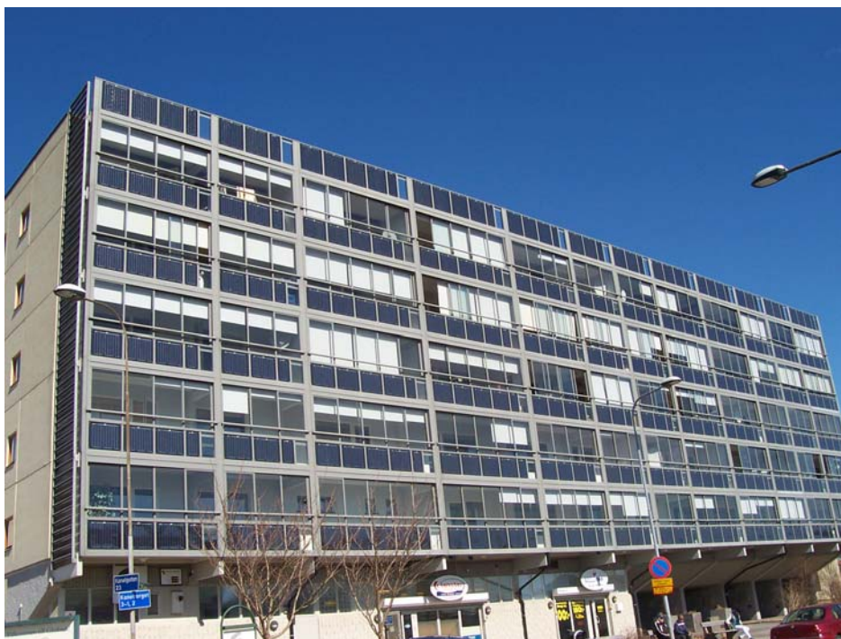
Figure 3.3 View of the PV plant integrated to the Kastanjgården building
