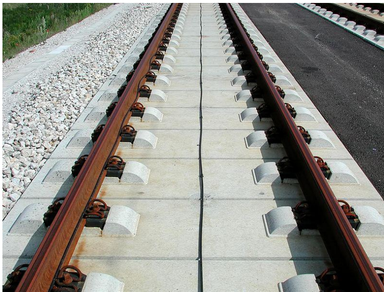
Figure 11 A slab track which is an example of a ballast free track solution (Wikipedia, 2013d).
