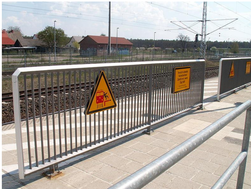
Figure 8 Example of fixed platform fences from Germany (Wikipedia, 2013a)
