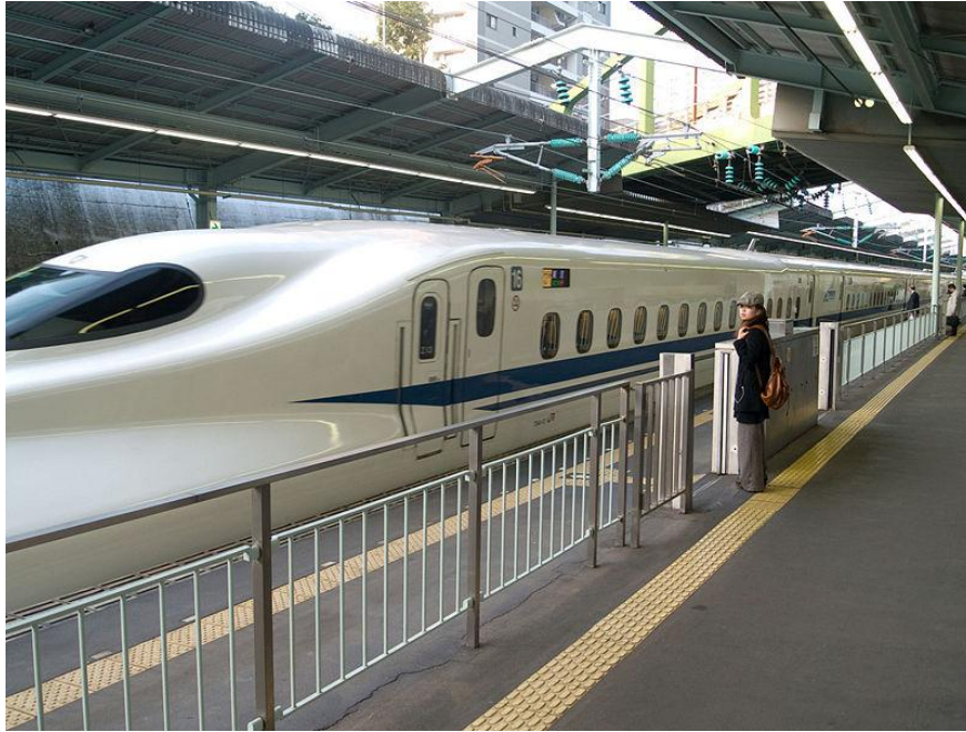
Figure 9 Platform fences with automatic gates in Japan. (Wikipedia, 2013b)
