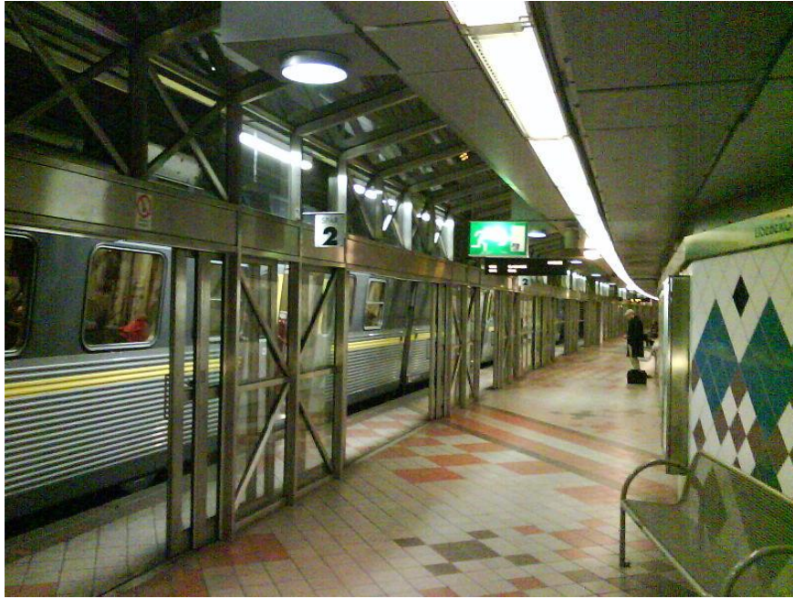
Figure 10 Example of Platform Screen Doors from Liseberg station in Göteborg (Wikipedia, 2013c)
