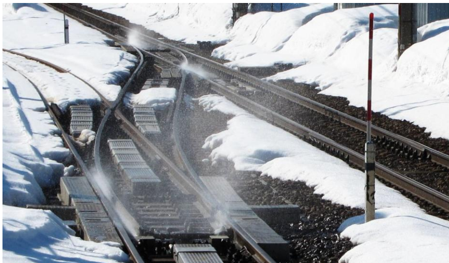
Figure 13 Hot water sprinklers that melt the snow at a switch (Ramböll, 2012).
