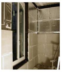
Figure 3.7Interior Insulation with VIPs in Zürich (Binz et al. 2005)
