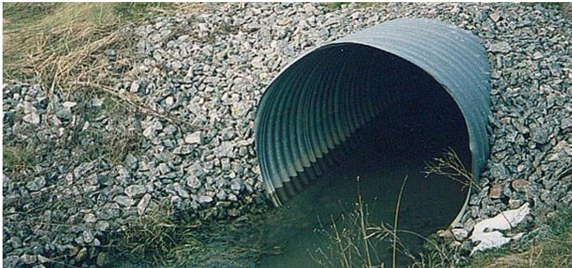
Picture 10 A good functioning culvert (ViaCon, 2010).
