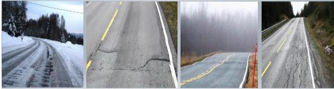
Picture 9 The possible damages occurring when there is frozen ground and without having any preventive solutions (Granlund, 2012).
