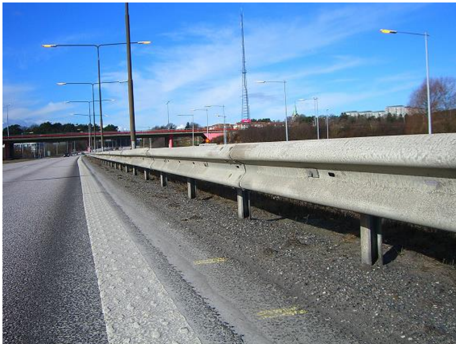
Picture 13 W-beam barrier (Karim, 2012)
