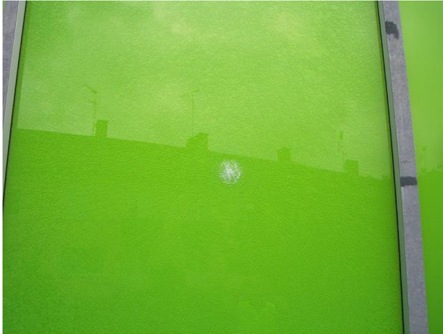
Picture 17 Illustration of broken green glass noise barriers at Kallebäck (Karim, 2012)
