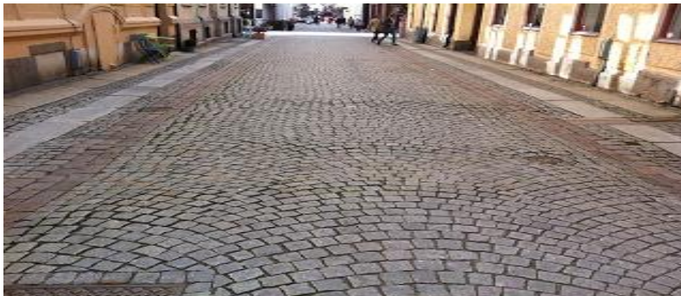
Picture 5 Settlings caused by heavy loads. The picture is taken in the city centre of Gothenburg (Bianchi, 2012).
