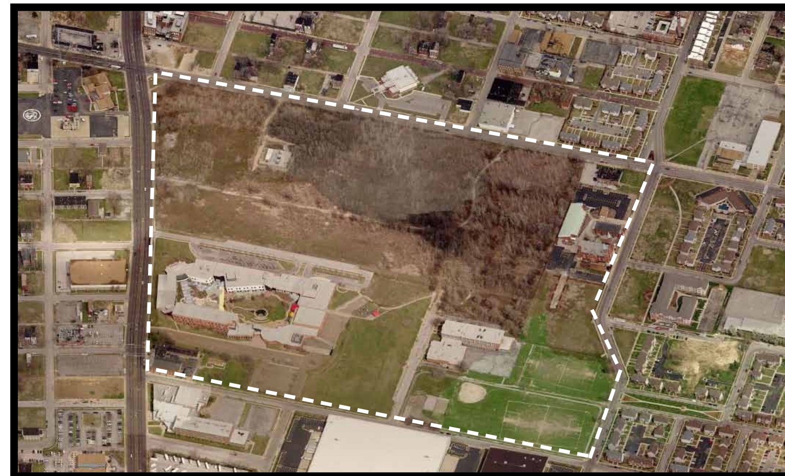
The Pruitt-Igoe site today, seen from South
