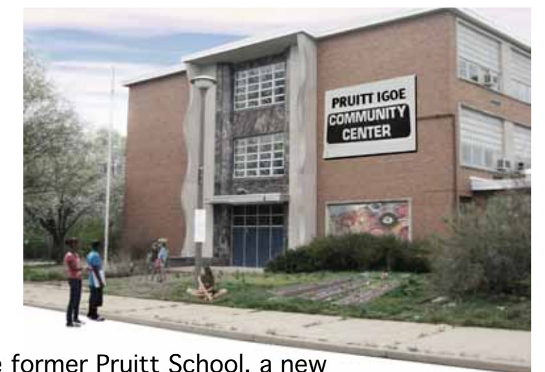
In the former Pruitt School, a new community center is established, providing space for local organizations and after-school activities.
