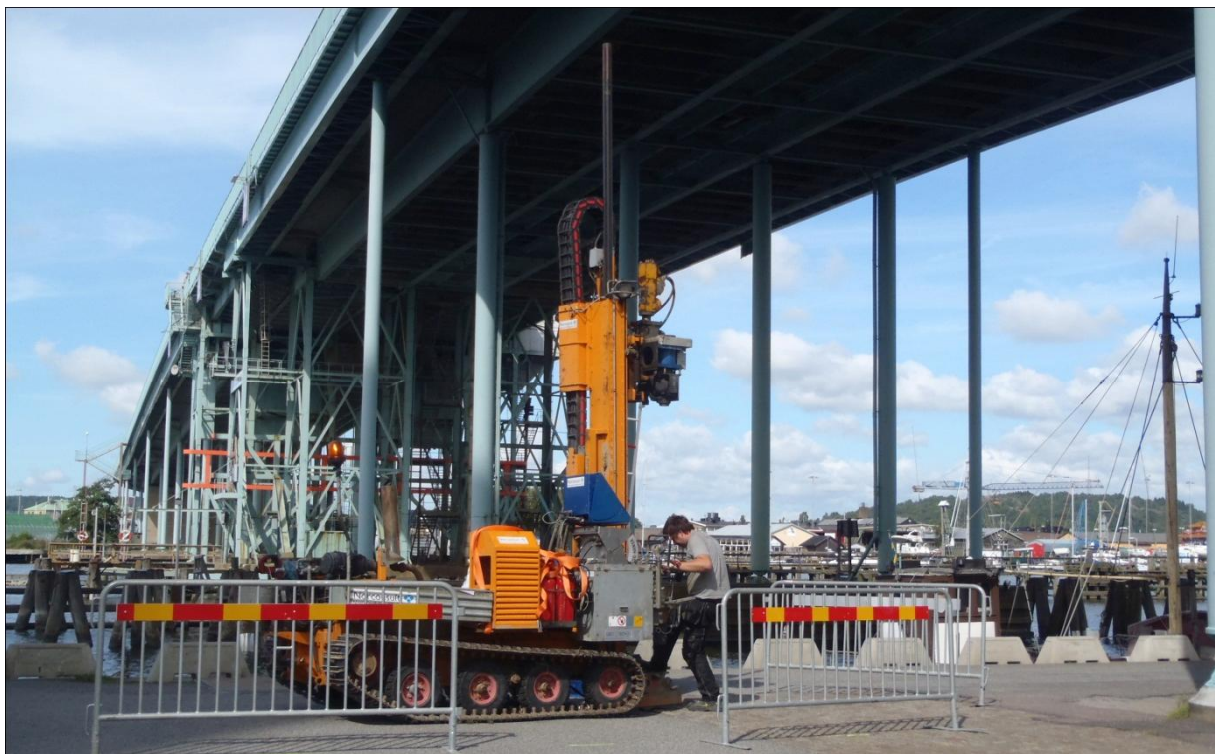
Figure 2.2: Soil sampling with a drilling rig, © Norconsult.
