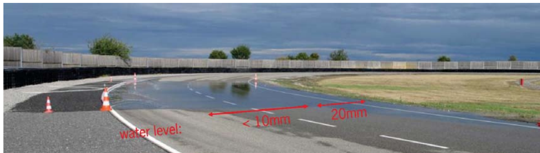
Fig. 3.17. Water drive trough.
