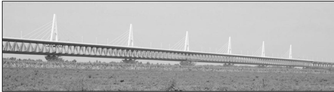
Figure 6 The main bridge of the Zhengzhou yellow river road-cum-railway bridge (Gao 2012).
