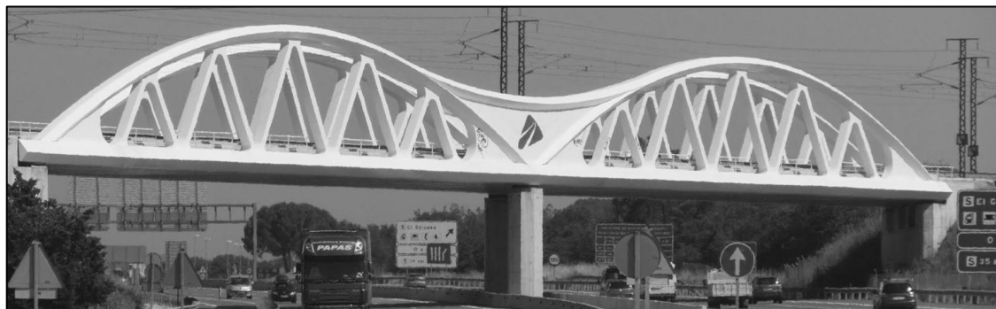
Figure 2 The Riudellots high speed line bridge (Skachkova 2012)
