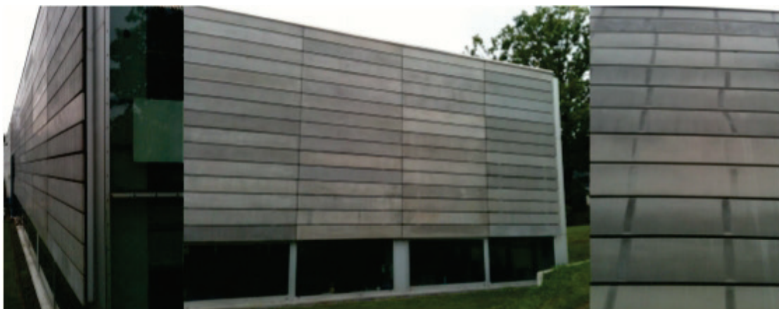
Figure 4.2 Curtain wall construction of the Structural Concrete Institute, RWTH Aachen University.
