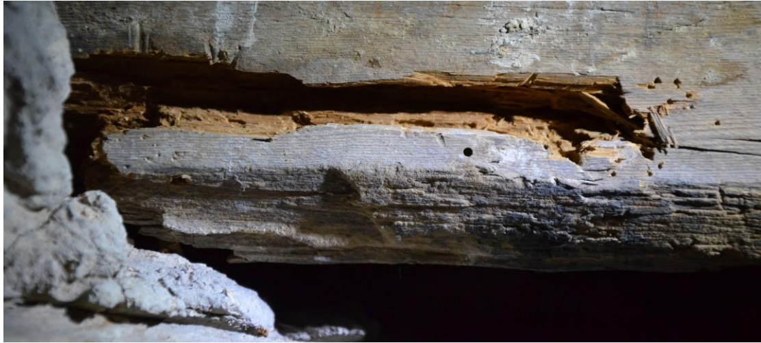
Figure 7.3 Damaged region at wall support of beam D in span 1 in lower floor. Several smooth holes (one visible near the centre of the image) raised concern about eventual damage close to the surface and the bottom face. After probing with a screwdriver the damage was revealed and explained as an insect attack.
