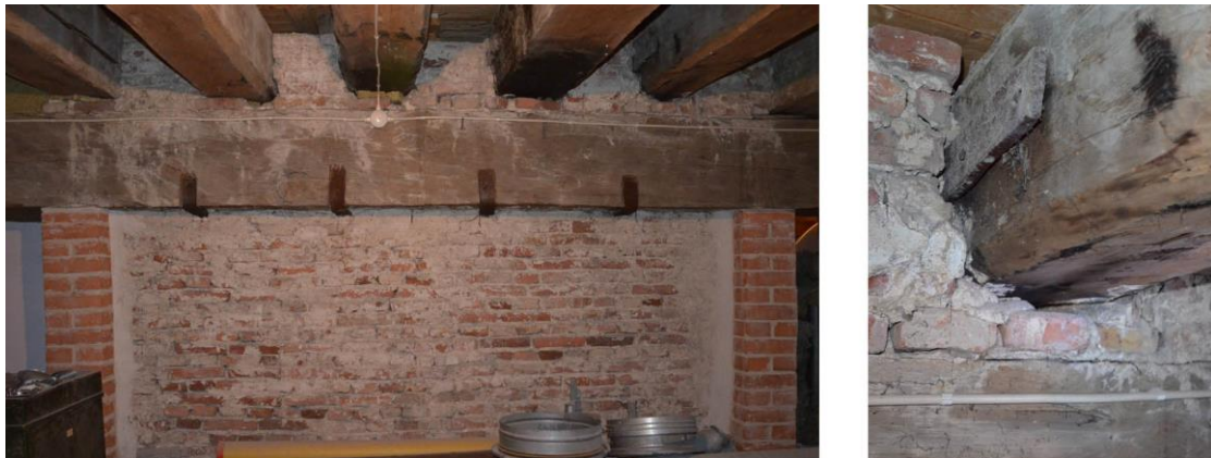
Figure 8.1 Photography of primary beam 1 in first artillery floor, supported by the masonry structure (Left) close up view of the anchorage detail for the rightmost secondary beam K (Right), cf. Figure 8.2.
