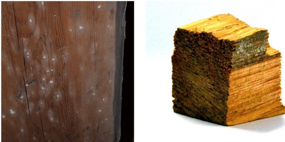
Figure 7.2 White specks and discolouration in the lower floor (Left) and piece from the removed part of beam P showing damage on the earlywood and fungal growth (grey spots, right).
