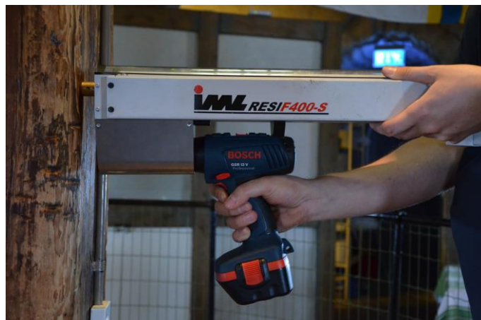
Figure 7.18 Electrical resistance drilling device driven perpendicular to the timber surface of a column during the in-situ testing.
