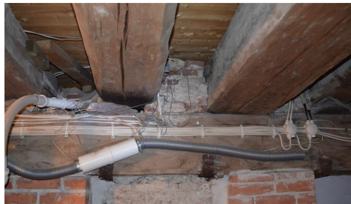
Figure 8.6 Middle support for primary beam 2 in the lower floor.
