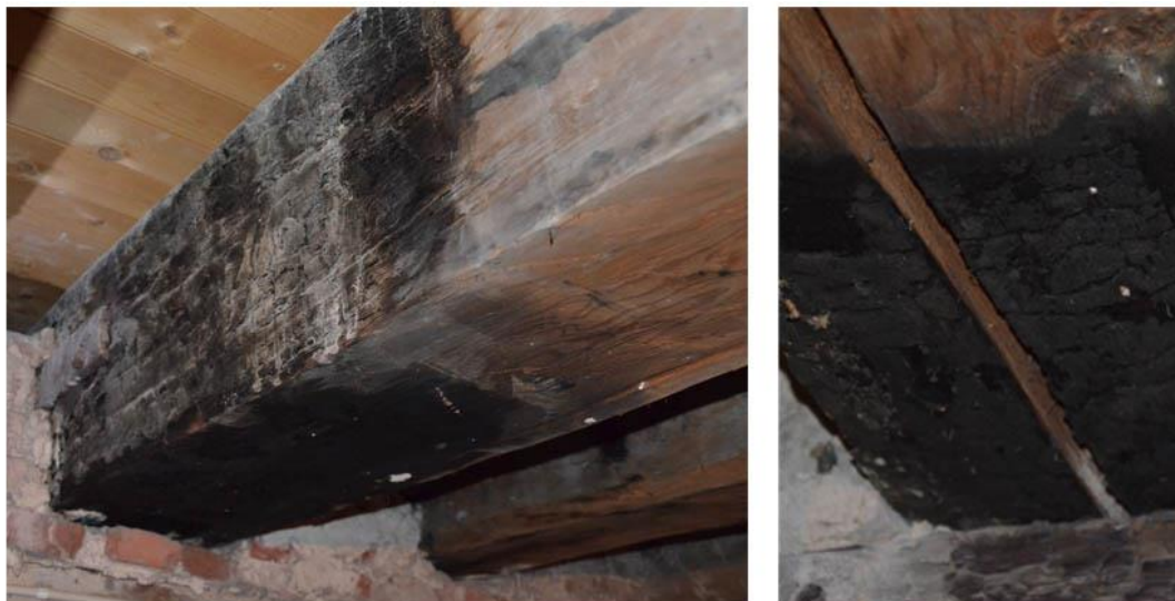
Figure 7.1 One of several charred beam edges at supports (Left) and the thickness of the charring is revealed by the crack (Right).
