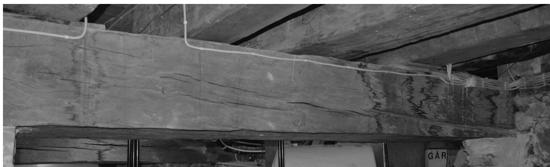
Figure 2.4 Example of discolouration in Skansen Lejonet on a primary beam (to the right).
