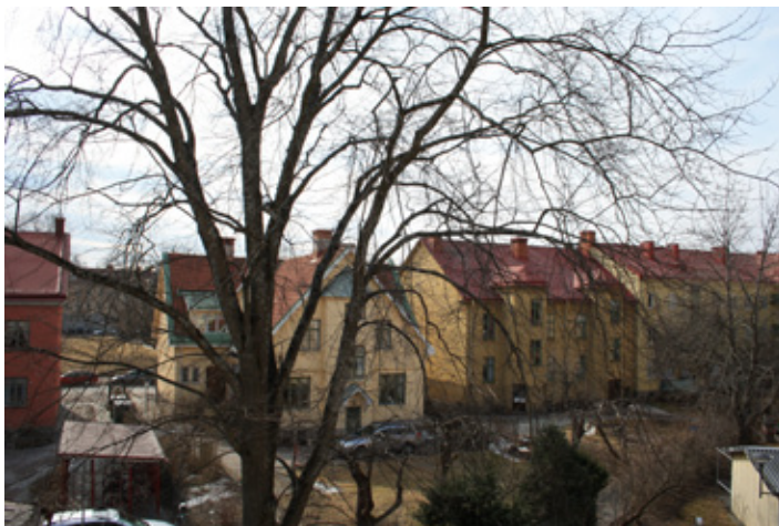
8. View on the courtyard of the block Törnrosen
