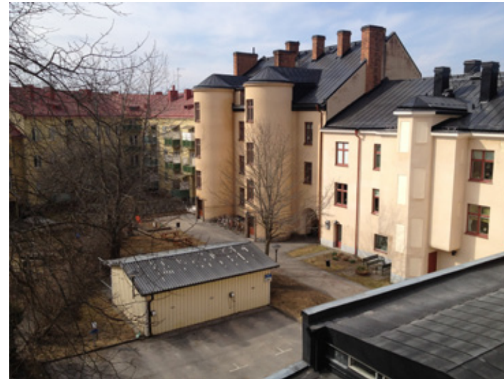
4. Overlooking part of the 1980s addition (to the right) and the neighbouring courtyard
