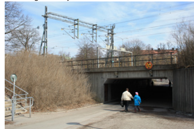
A tunnel under the railway was built in the 1970s connecting Väster with the city centre
