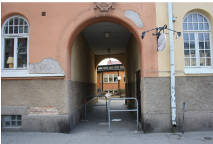
9. Entering the courtyard of IMK
