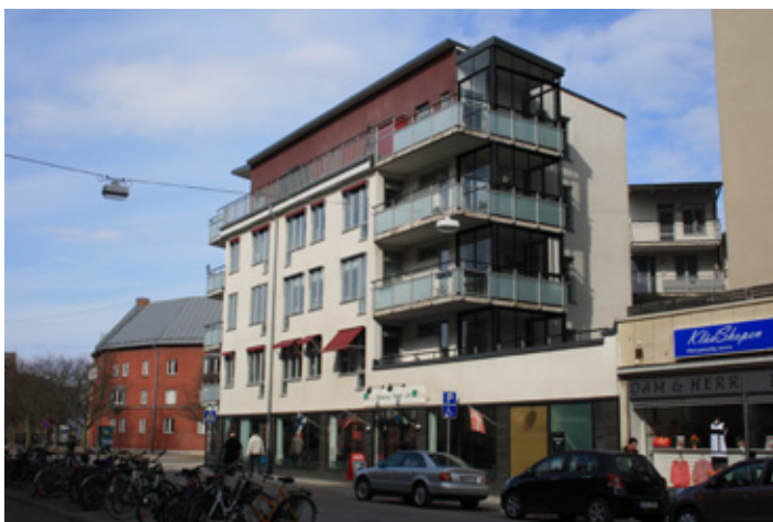
C. This building is a later addition in the same scale as the rest of the block. Also with a restaurant in the first floor.
