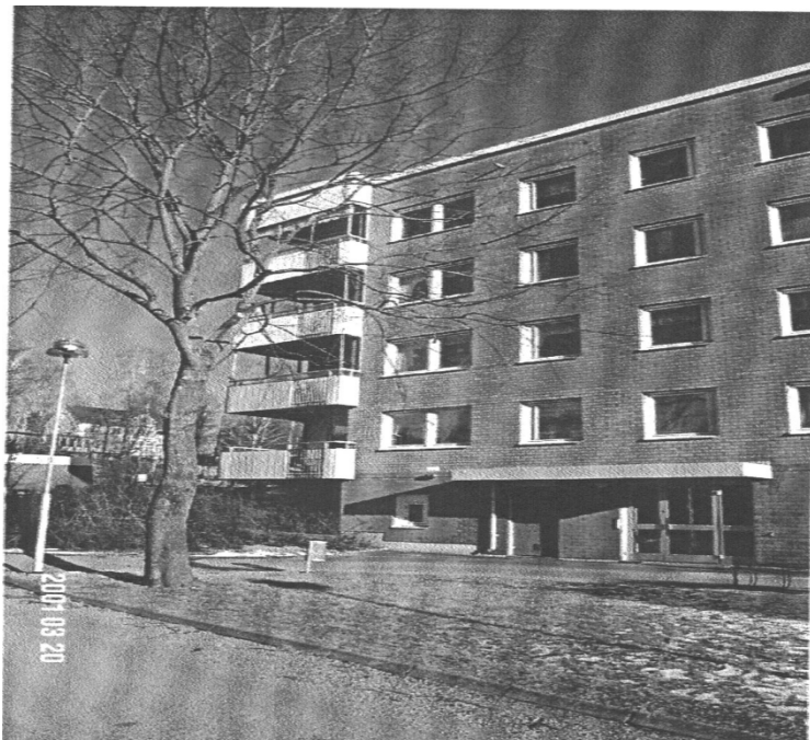
Figure 16 Facade of the test building, facing towards NW.
