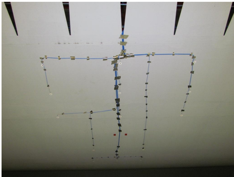
Figure 4 Pressure measurement probes mounted in nozzle ceiling. Picture taken toward the flow direction.
