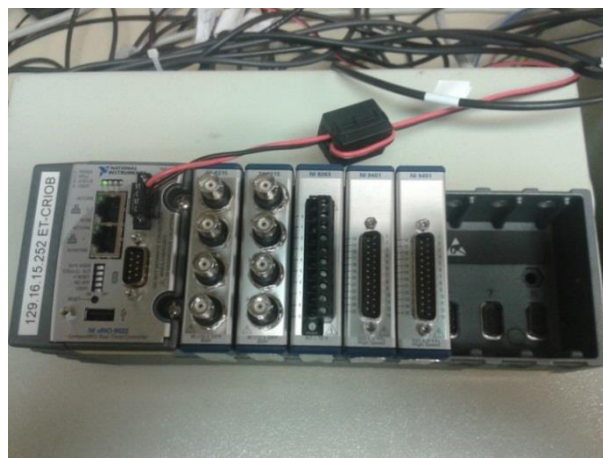
Figure 4.10: CRIO 9022 controller with the used modules.
