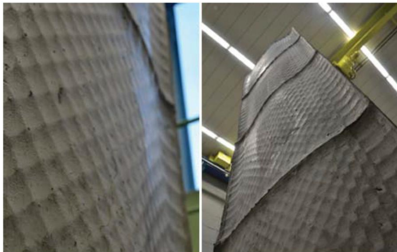
Figure. 31: Surface finish detail produced by moulded wax formwork
