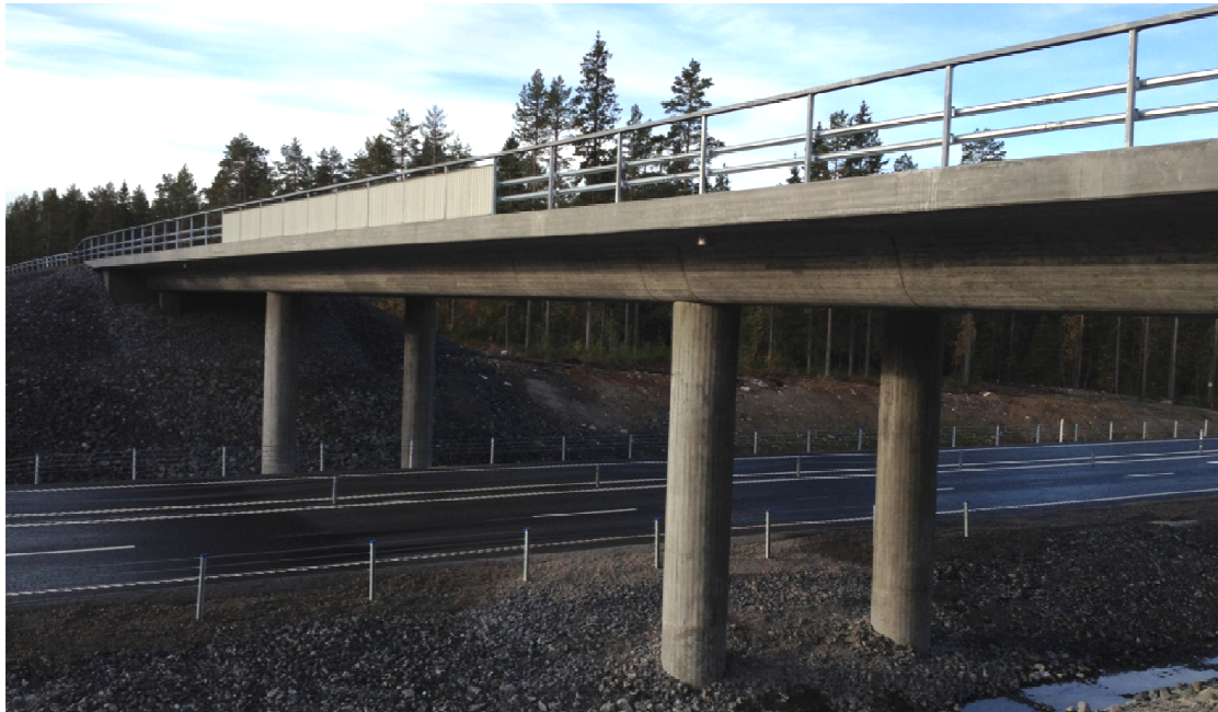
Figure 6.1. Example of a three-span double-beam bridge. The geometry of the studied bridge is loosely based on this one.
