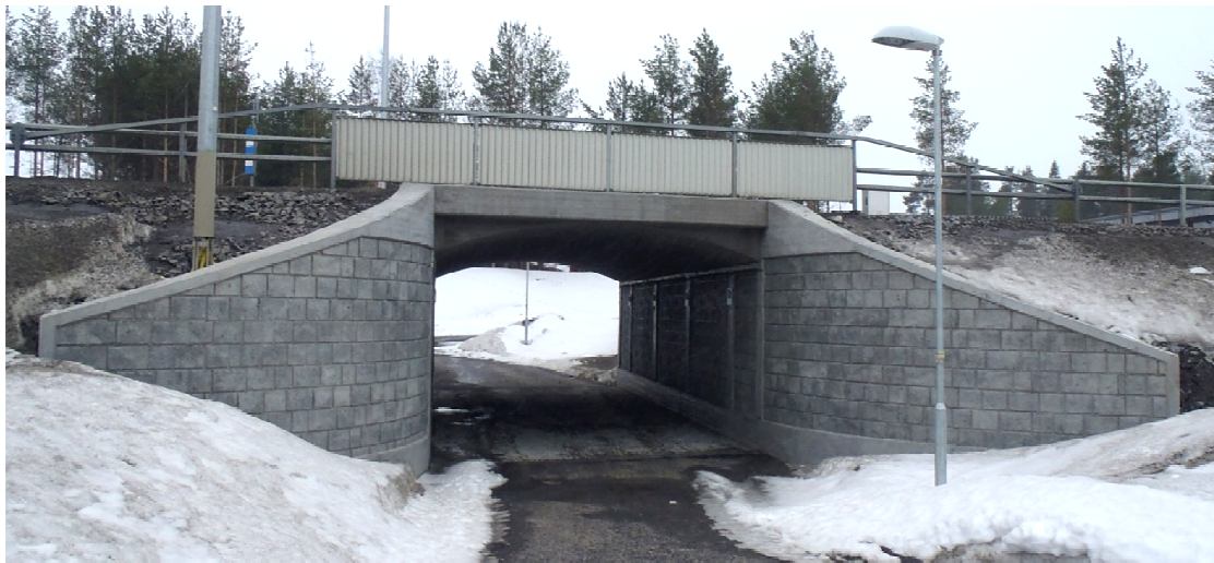
Figure 5.1. Example of an integral slab frame bridge with curved wing walls and circularly haunched bridge deck. The geometry of the studied bridge is loosely based on this one, where a swedish national highway crosses a walk- and bicycle path.
