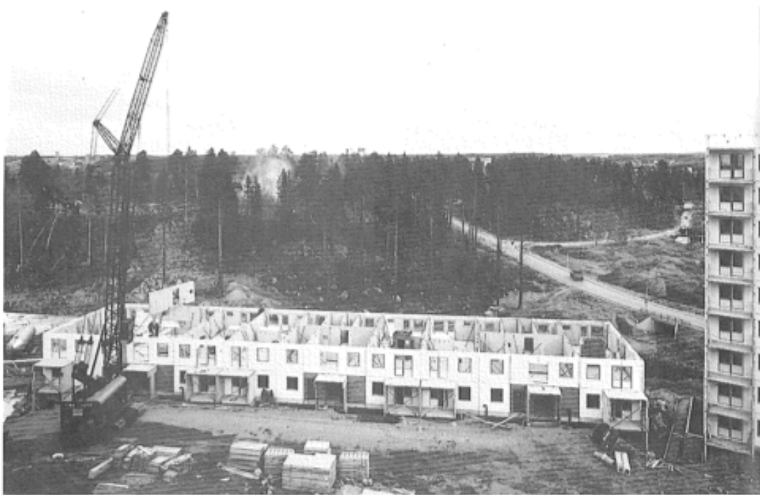
Figure 4 Picture of a typical house built with prefabricated elements (Vidén & Lundahl 1992)
