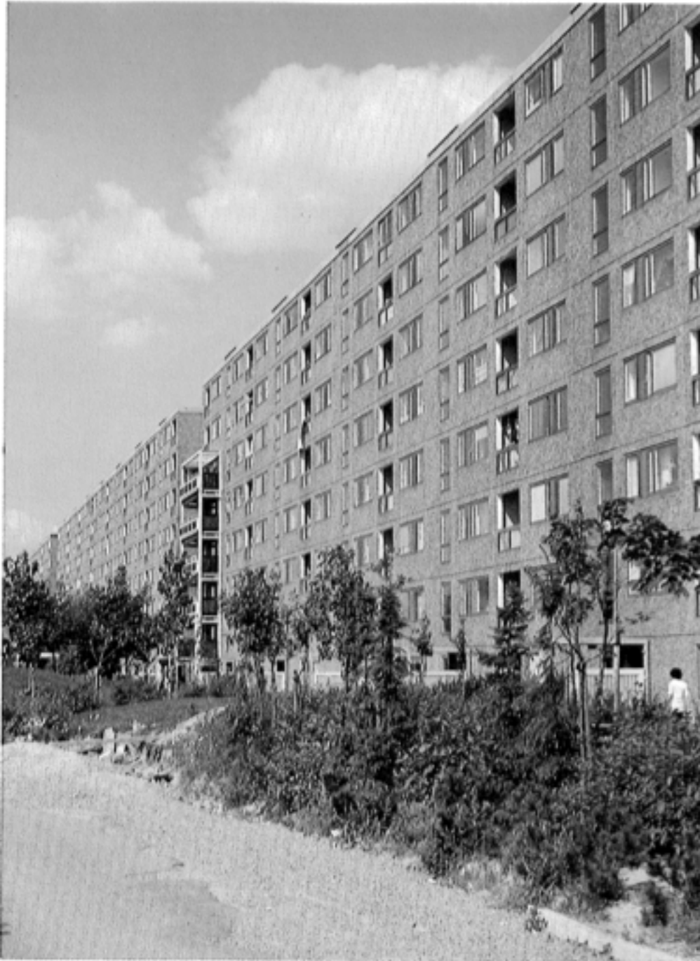
Figure 7 Typical higher slab-block houses, Gothenburg (Björk, Kallstenius & Reppen 1992)
