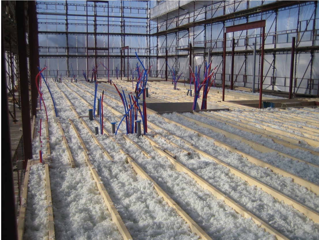
Figure 16 A wooden beam grid that lies on top of a steel grid (the steel grid is not visible), Fredslyckan.
