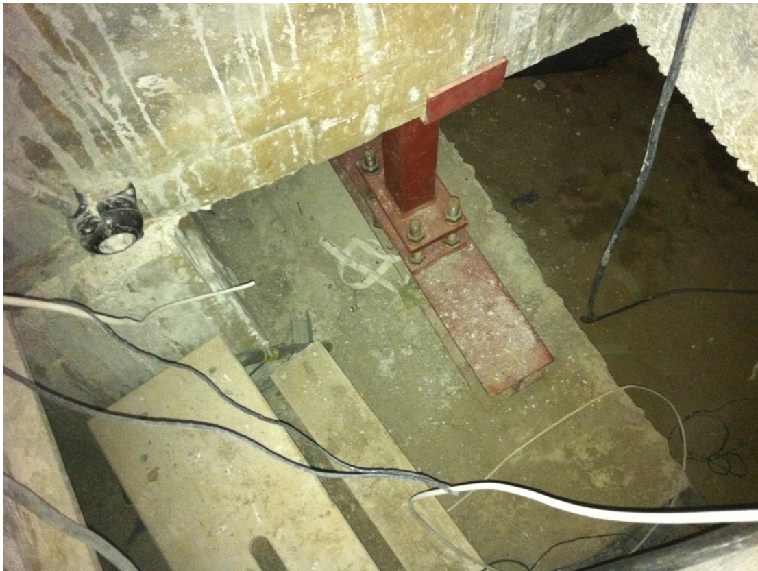
Figure 12 Steel beam supports at a plinth foundation, Fredslyckan
