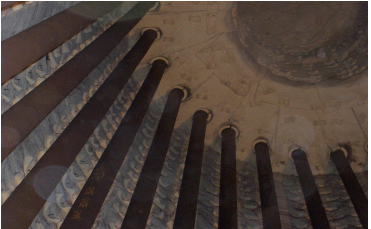
Figure 5: Picture taken inside the Bohus reformer furnace. The tubes are arranged in a circle inside the walls. The outlet for the flue gases is at the top of the reformer.
