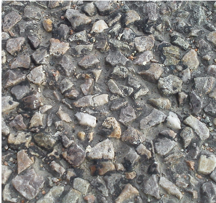
Figure A.26.: Photo of the measured porous asphalt surface layer. The inner diameter of the sealant circle is 80 mm.
