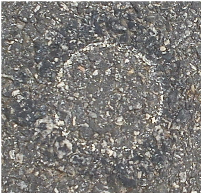
Figure A.25.: Photo of the measured regular road surface layer. The inner diameter of the sealant circle is 80 mm.
