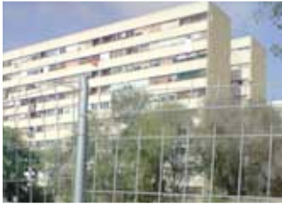
La Mina, Barcelona, Spain
