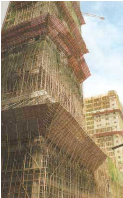
Bamboo used for scaffolding Source: Bambus - RWTH Aachen 2002
