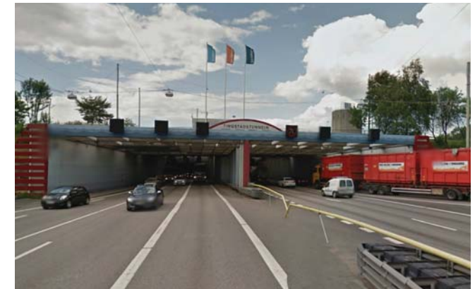
Figure 42 The entrance of Tingstadstunneln (Google, 2013)
