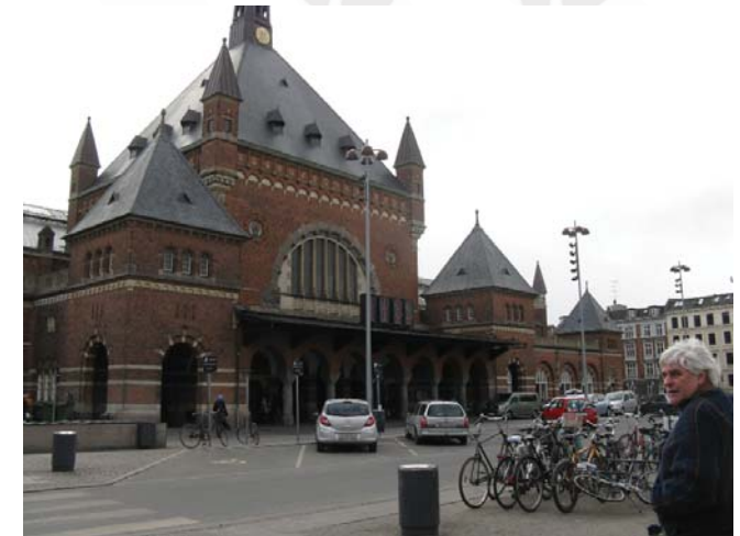
Figure 38 Copenhagen Central station
