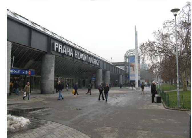
Figure 31 Prague Main Train station, new entrance
