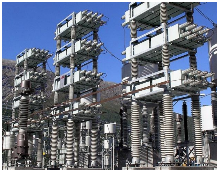
Fig.2.4. Substation capacitors from ABB. Image courtesy of ABB Power Capacitors
