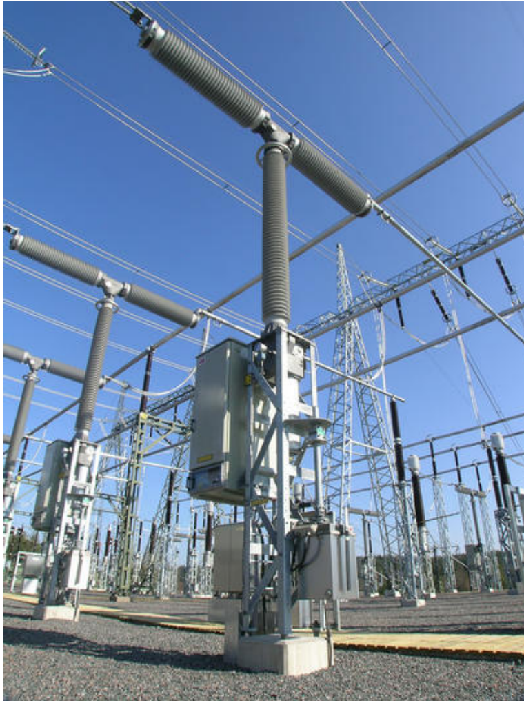
Fig. 2.10 HVL Combined Disconnecting Circuit Breaker (courtesy to ABB)
