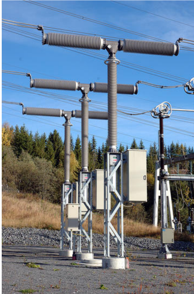
Fig. 2.9 HPL B for outdoor installation (courtesy to ABB)
