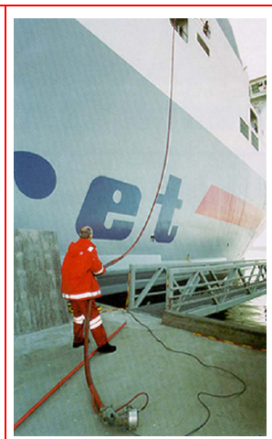
Figure B7 A single main cable for the power supply and manoeuvre is all that is needed to connect the ship.
