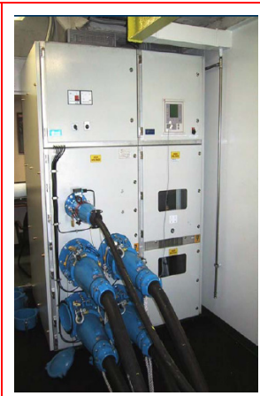
Figure B24 The connection box on the ship connecting 4 power connectors, 1 neutral connection and the cables for controlling.
