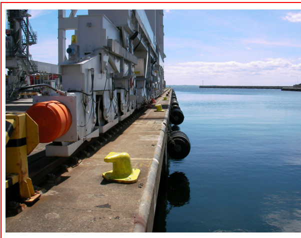
Figure C33 The free space between the crane and the quay-side is limited, approximately 1 meter.
