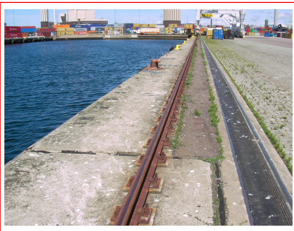
Figure C34 Cranes operate on fixed rails and require the full range of the quay.
