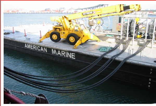
Figure B15 A barge with the transformer and a cable reel is moored at the stern of the container vessel. Nine heavy cables are hoisted into position using a crane.
