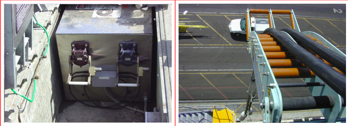
Figure B19 The electrical vault with two connectors located in the side of the quay.
