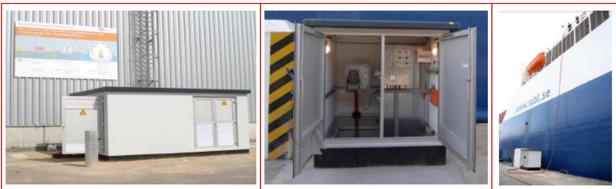
Figure B13 Cabinet with a 6.6 kV/50 Hz outlet enabling power to be obtained from the berth.
