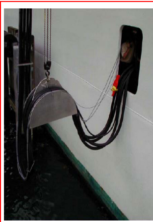
Figure B23 Four cables are used for the electric power connection and they're hoisted into position by the cable arrangement system.
