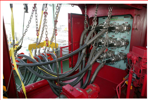
Figure B16 The 9 cables are connected to the vessel connection box.
