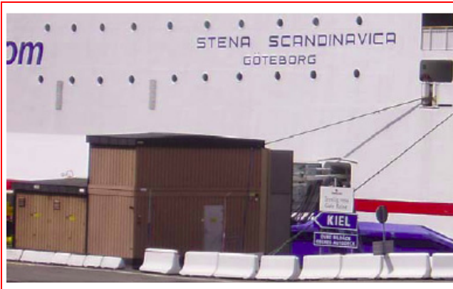
Figure B3 The first shore-connection in Port of Göteborg, installed in 1989 at the Kiel terminal. The building in the picture includes the transformer and cable arrangement equipment.
