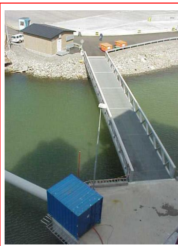
Figure B5 The first high voltage installation in Port of Göteborg. The building in the top left contains a transformer and switchgears. The blue container building is the connection point.
