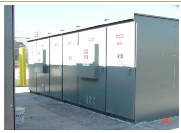
Figure B18 Main and Metering Equipment (6.6 kV)
