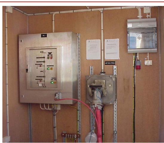
Figure B6 The figure illustrates the interior of the blue 9ft container building. The main cable is connected to the outlet and, the manoeuvre cable is connected to the control panel where the person performing this action has an overview of the whole system.
