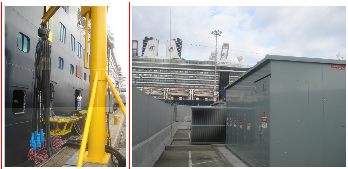
Figure B27 Cables are hoisted into position using a gantry. Each cable contains three cores (L1,L2,L3) and can carry 500 A per phase by 11 kV.
