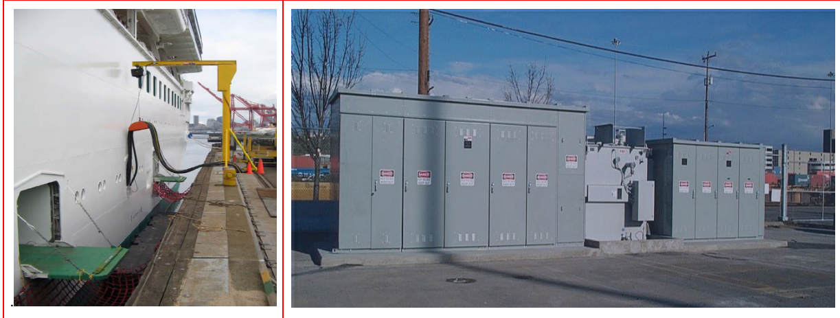
Figure B25 Cables are hoisted into position using a gantry.
