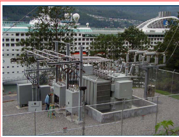
Figure B22 A dual-voltage transformer is used to step down the voltage from the local power grid to 6.6 kV or 11 kV.
