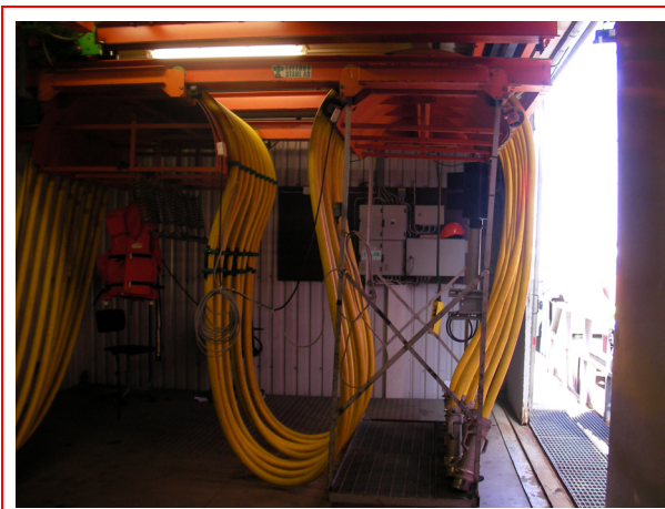
Figure B8 The cable arrangement building next to the berth for the first installation in 1985.
