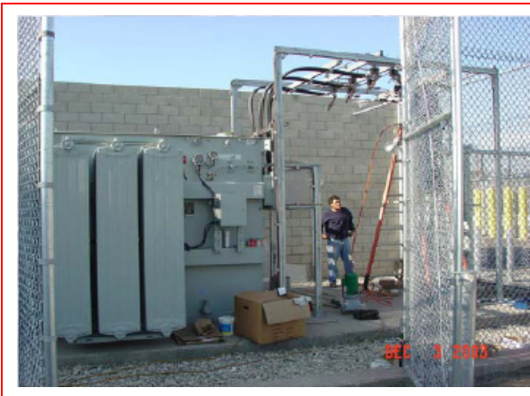
Figure B17 The utility transformer (34.5/6.6 kV 7.5 MVA) located on the harbour site.
