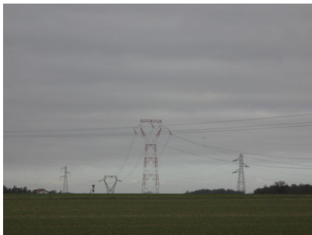
Fig.4: Picture of a high voltage line (Source : Encis wind)
