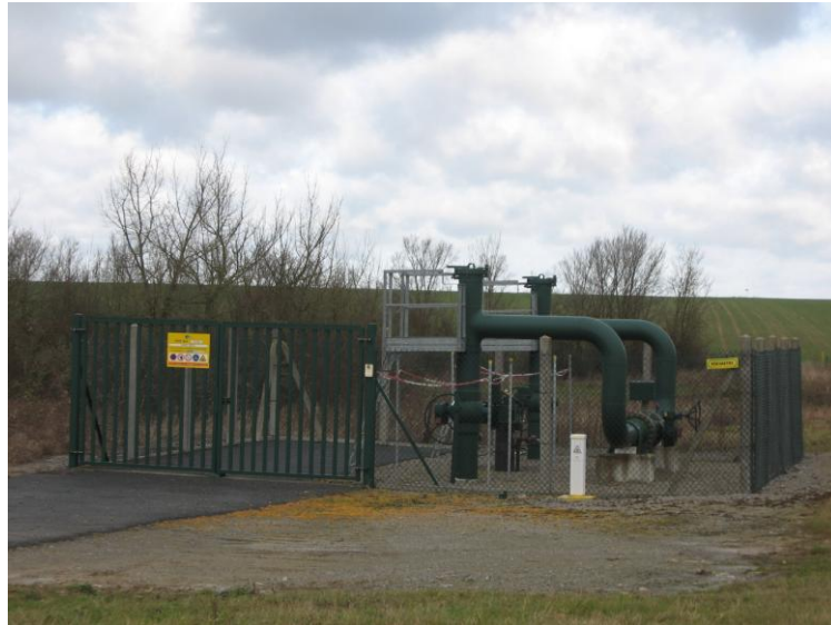
Fig.6: Picture of a gas expansion station (source: Encis Wind)
