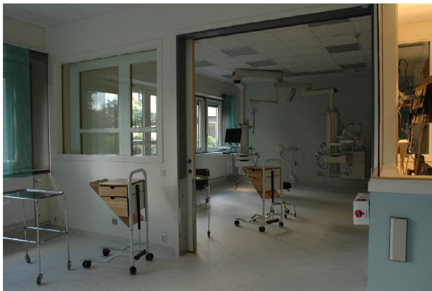
Figure 54 - NÄL ICU - Sliding Door Between Patient Rooms (Ek 2012e)
