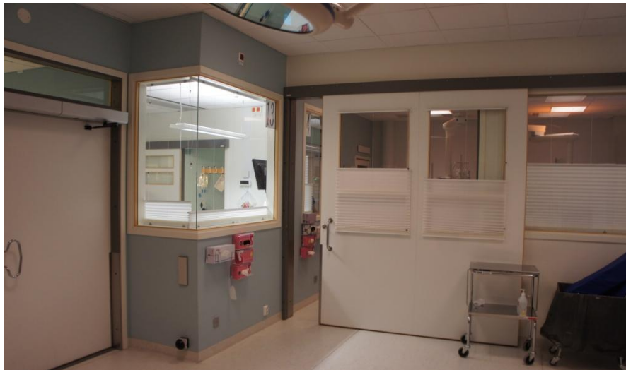
Figure 5 - ICU 3, from left: room entry door, documentation room window, and sliding door connecting two patient rooms
