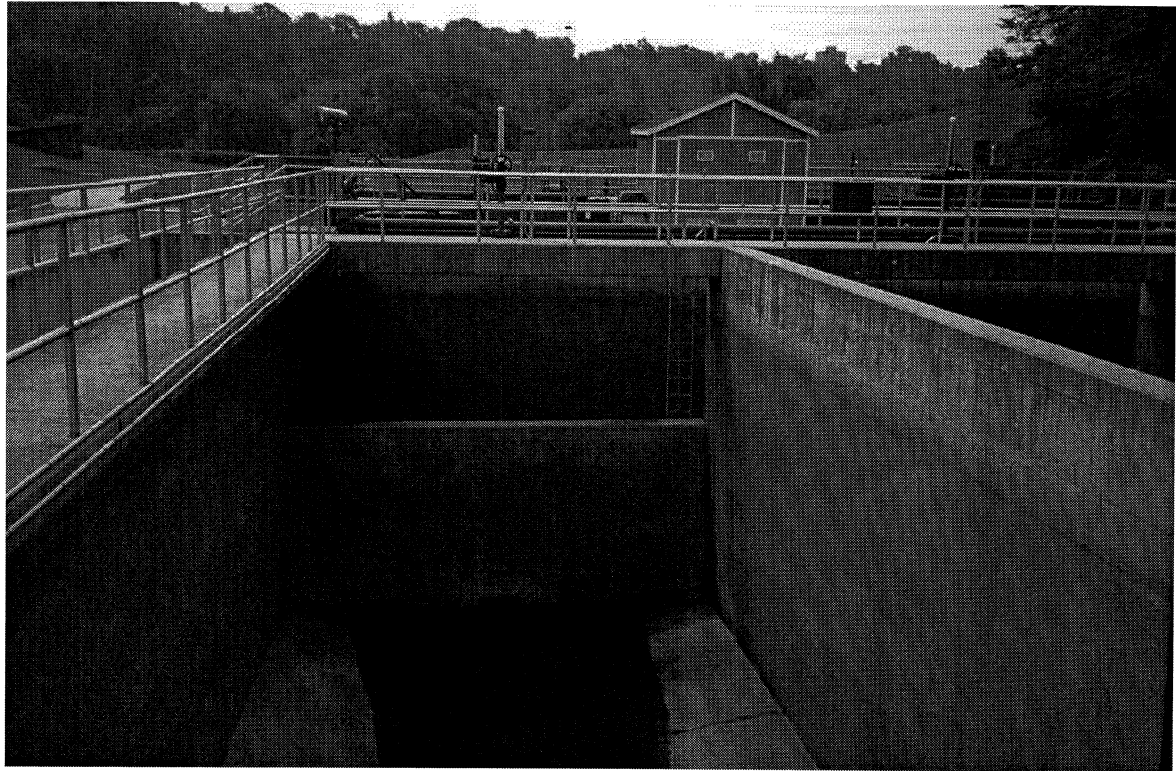
Fig. 5.4.3. Dry Tank 1 towards inlet. (Photo by Quintin Rochford)
