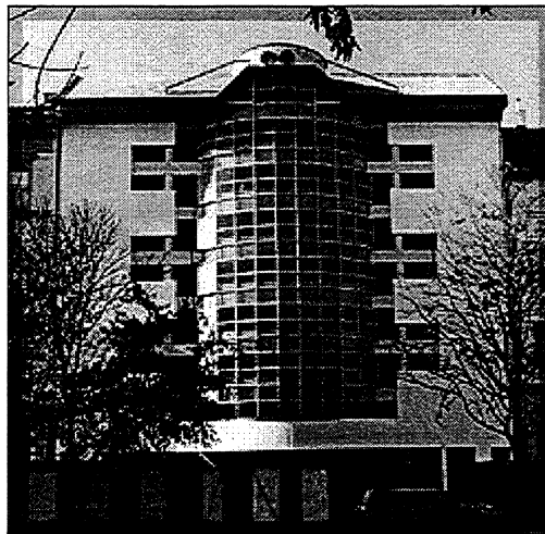
Figure 12: Multilevel parking house – Nyár street
