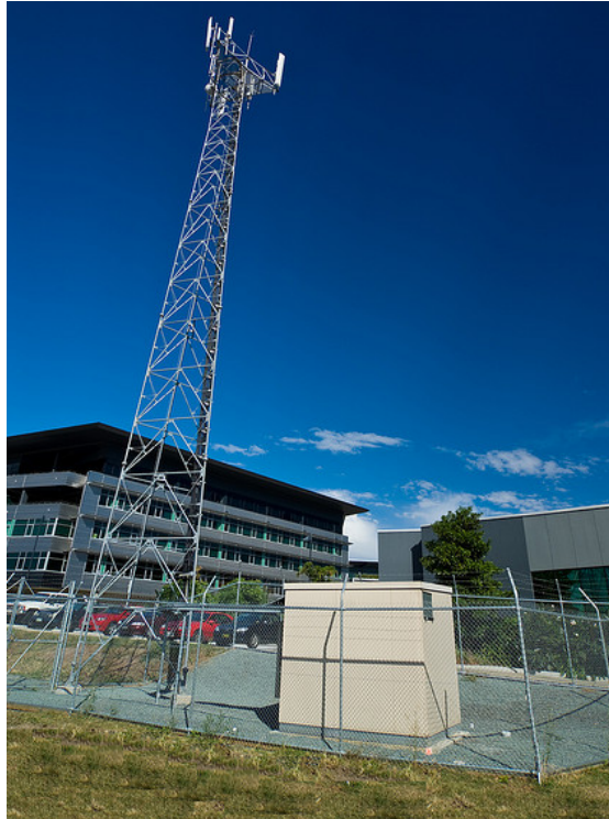
Figure 1.1: High baseband tower including cabinet
