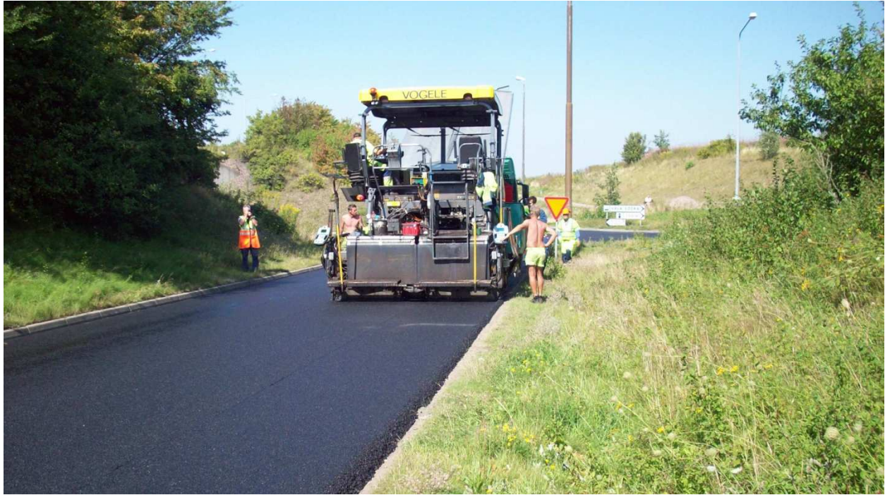
Figure 6 – In the paving process of warm mix asphalt with Rediset, the amount of fumes are reduced.
