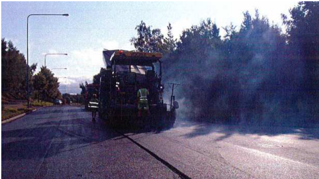
Figure 5 – In the paving process of hot mix asphalt, the amount of fumes are visible.
