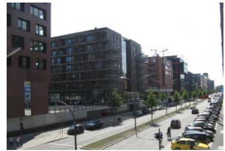
Figure 33. Buildings sit on elevated plinths Source: Woudstra, 2010
