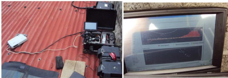
Figure 25. Data processing unit installed at Cristo Rey
