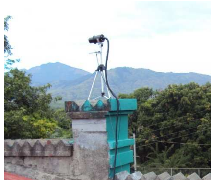
Figure 22. Installation at Cristo Rey site
