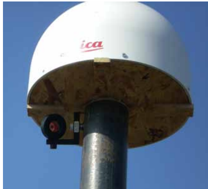
(b) Prism mounting at the top of the mast
