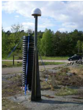
(a) Mast construction
