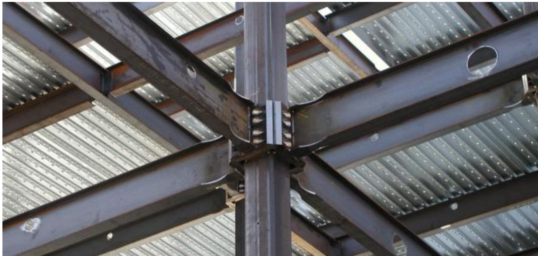
Figure 4-3 Connection Collar (JJeong, 2011)
