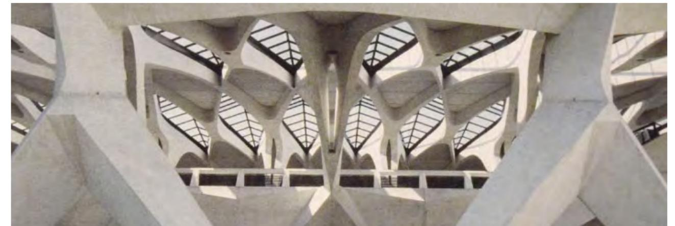
Fig. 15, Complex weight-bearing system, Gare TGV de Lyon, France
