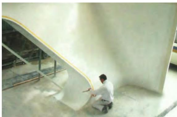
Fig. 23, Mineral foam, external insulation sawed and rasped in to shape in the construction of Casa Villa, Germany
