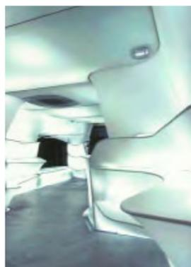
Fig. 21, PVC spanned across steel bars, United bamboo Store, Tokyo
