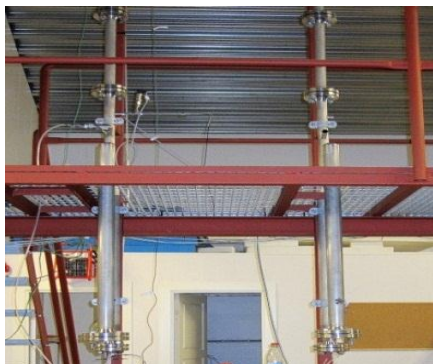
Figure 18 Absorber and Desorber
