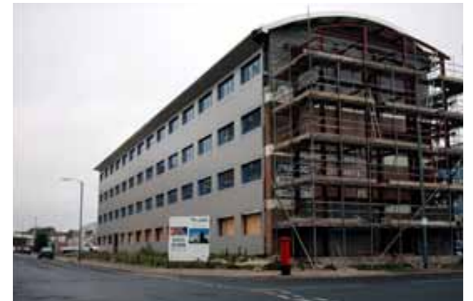
Intec House, Brighton - During Refurbishment
