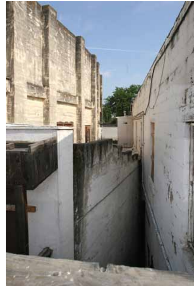
Before Existing link between two buildings
