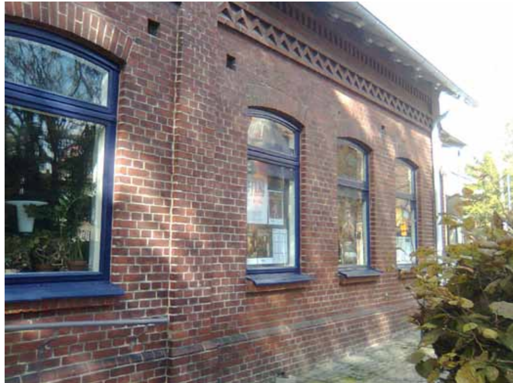
Windows in this part of building(administration) saved and just repaired ,Bricks in facade have been kept from original building and just renovated some parts,but new roof added to building
