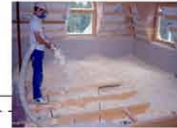
CELLULOSE FIBER INSULATION (Ekofiber AB, Kolinge, southern Sweden \lambda=0.039 W/mk
