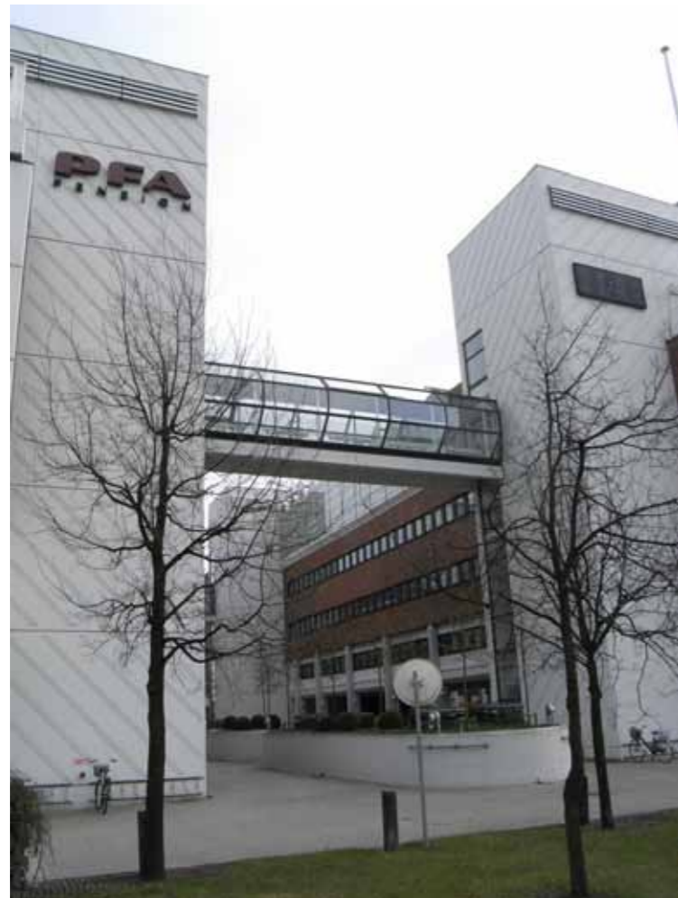
PFA pension office one of the new constructions in Nordhavn
