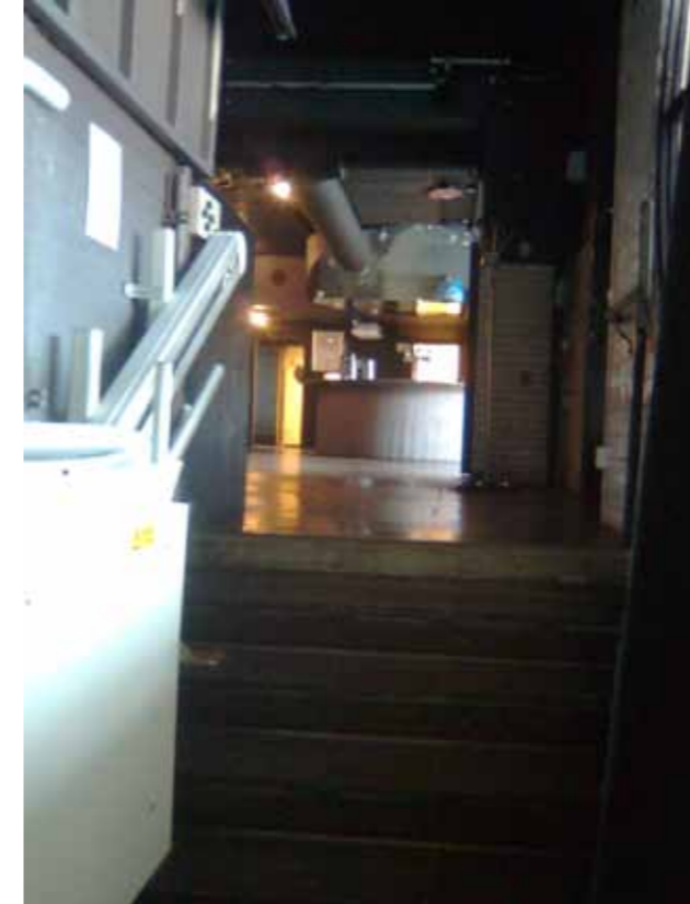
Corridor between main entrance and Cafe ,different levels need a lift for disables
