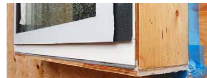
Proper air tightening can significantly reduce heating and cooling costs. On this picture the gap between the wall and the window has been sealed.
