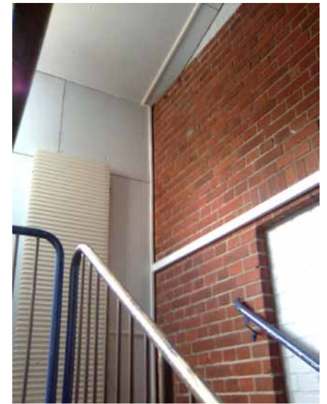
Staircase to back stage and connection between new and old brick walls
