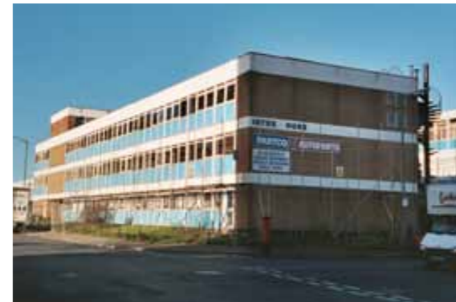
Intec House, Brighton - Before Refurbishment
