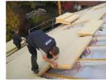
GUTEX ULTRATHERM Insulating, Rain tight, woodfiber \lambda=0.043 W/mk
