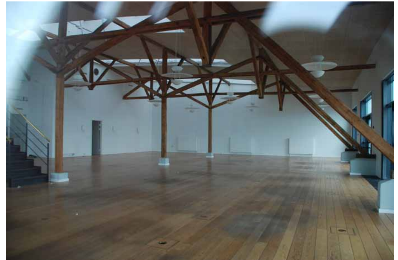
This industrial building renovated and re used and now it is an exhibition for one of the famous Danish furniture factories.It is located near the project site.
