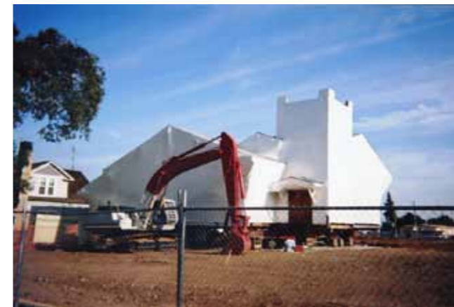
Before Old church on a wheel to move new site
