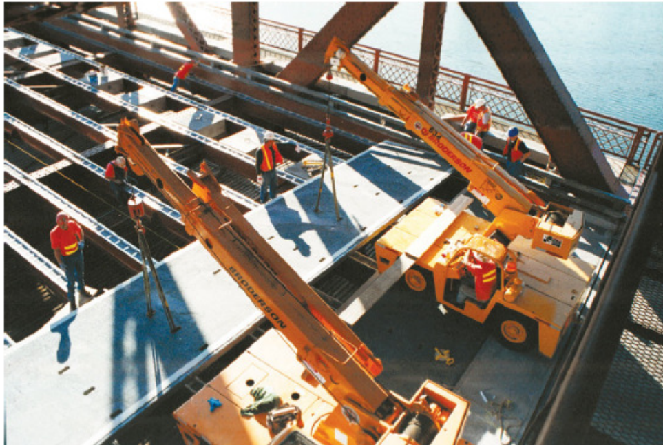
Figure 2.4: FRP deck panels were set in place with dual forklifts. (Matt Sams)
