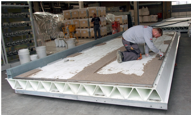
Figure 2.7: Preparation work for rapid assembly. (Fiberline)
