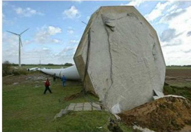
Figure 2.2 A collapsed power plant due to loss of equilibrium SMAG (2011).
