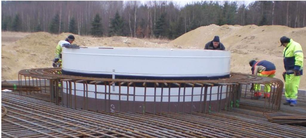
Figure 5.4 The anchor ring in the reference case during reinforcement installation.
