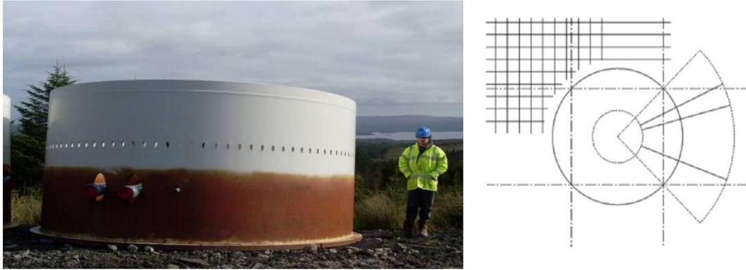
Figure 6.8 Left: Example of an anchor ring with holes where star reinforcement is placed. ESB International (2010). Right: Principle arrangement of star reinforcement.
