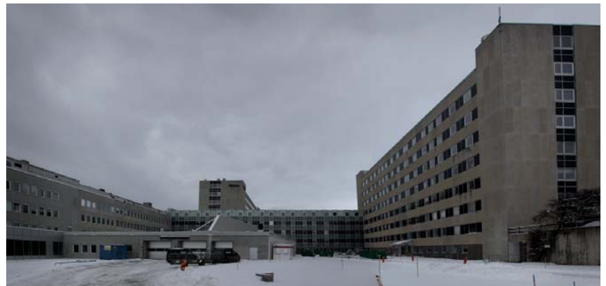
proposed site for new operation center
