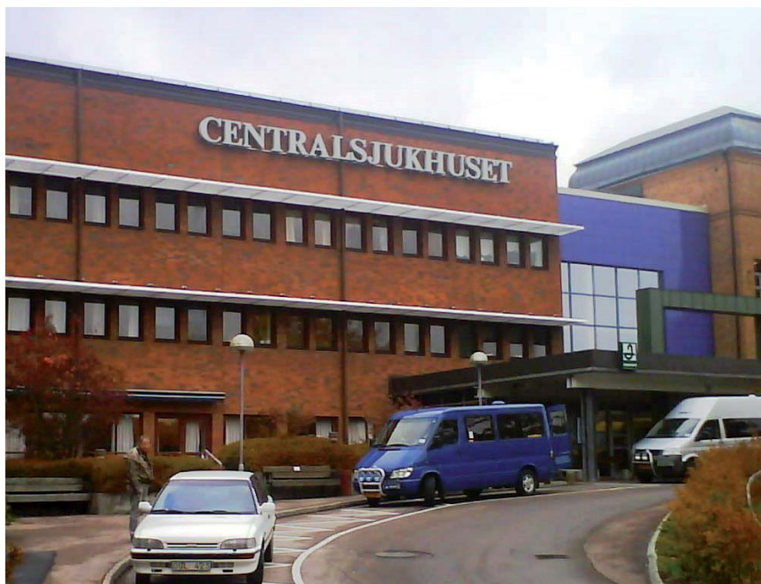
Karlsatd hospital Rebuilding of Operation room Sweco, 2012
