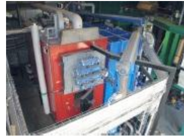
Figure 14: Boiler unit BIOAGRO
