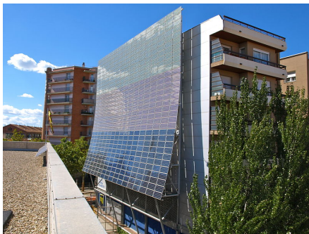
(a) Photovoltaic solar panels.
