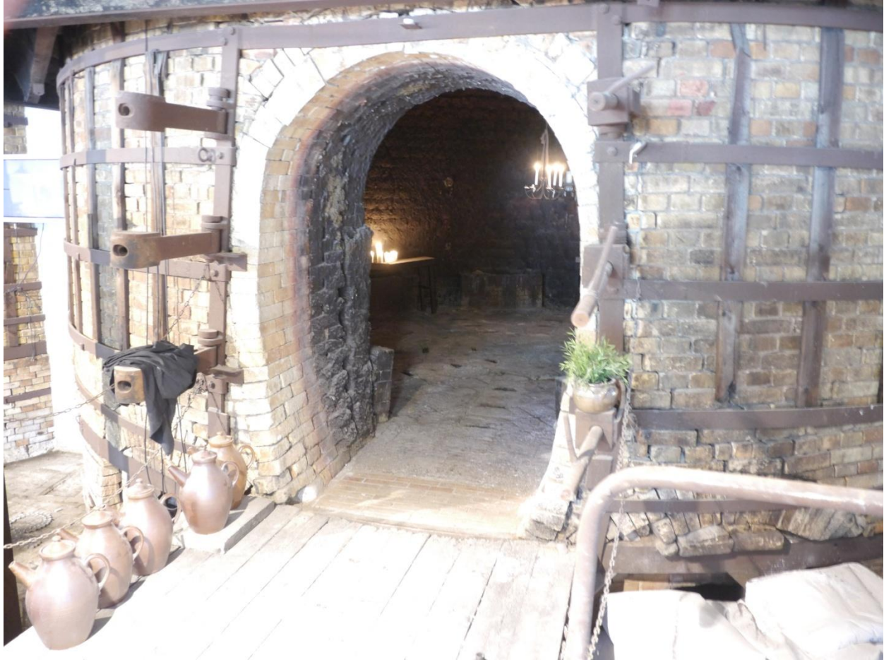
Figure 23 Picture of one of the old kiln is Höganäs, Sweden, where you can see the opening, one of the inlets and the outer walls
