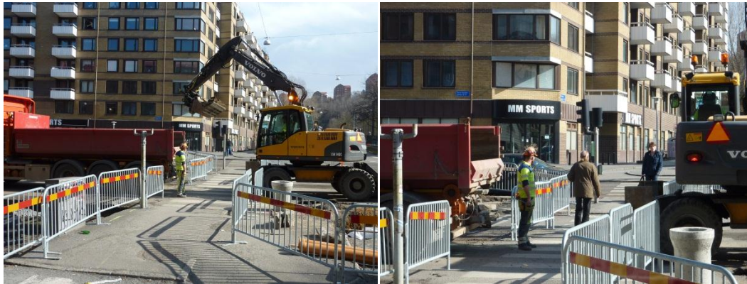
Figure 7. Excavator loading over the pedestrian crossing.
