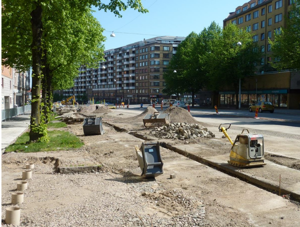
Figure 10. A closed off idle worksite.
