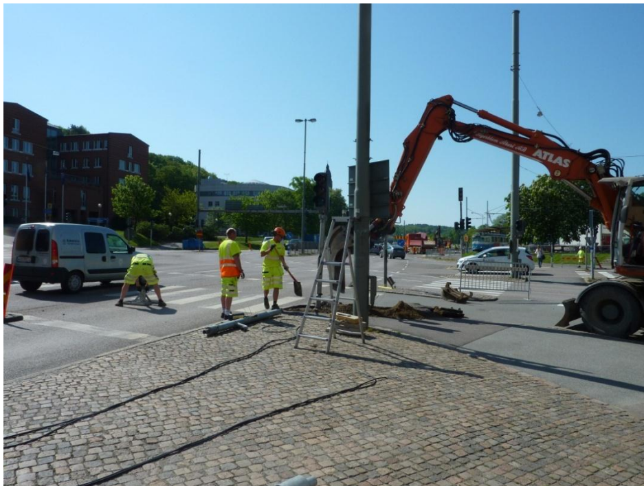
Figure 9. The construction worker to the left is working close to bypassing traffic.
