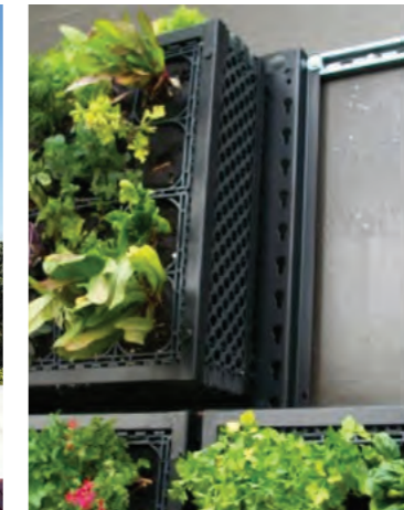
GREEN FACADE Module system for planting on the facade
