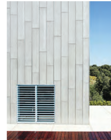
VIROC BOARDS Panels made from a mix of wood and cement.
