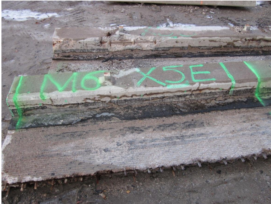
Figure 3.3 Edge beams and part of the slab after being sawn from the bridge.
